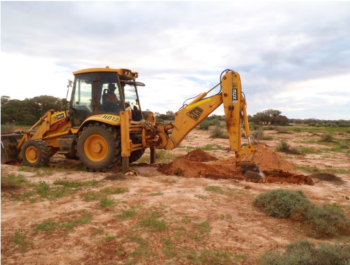
Plate 2.1: Excavation of investigation trenches
